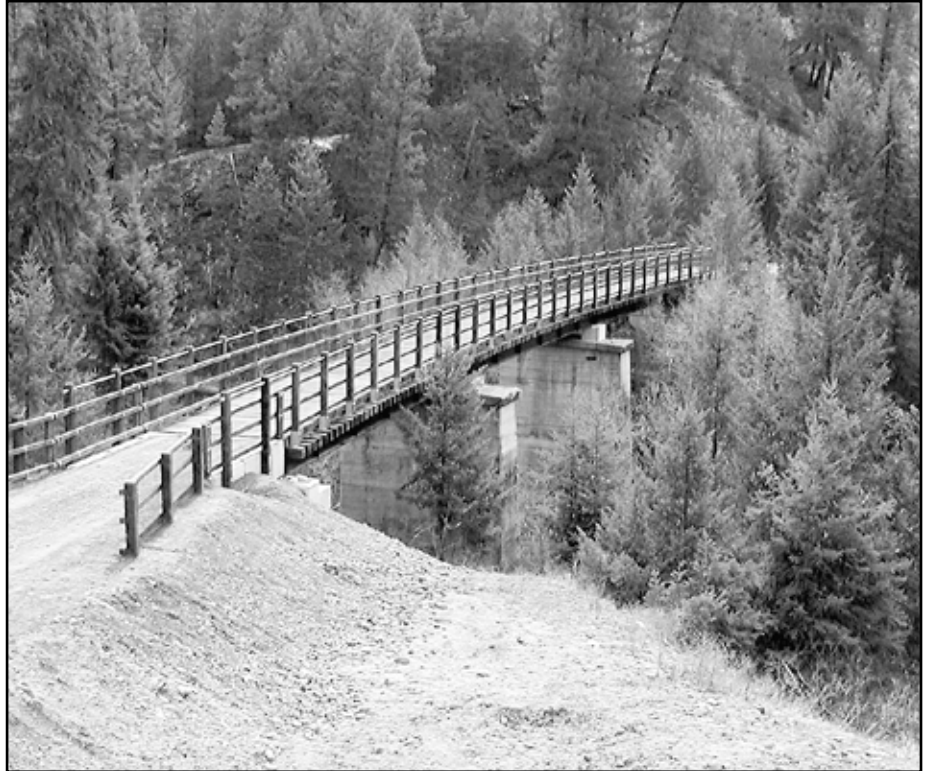
Bridge finished in Fall 2005 ~ Trout Creek #2, West of Faulder
