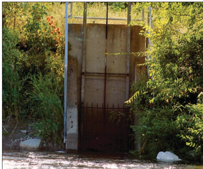
A valve for water regulation on the Okanagan River which supplies water for irrigation purposes
